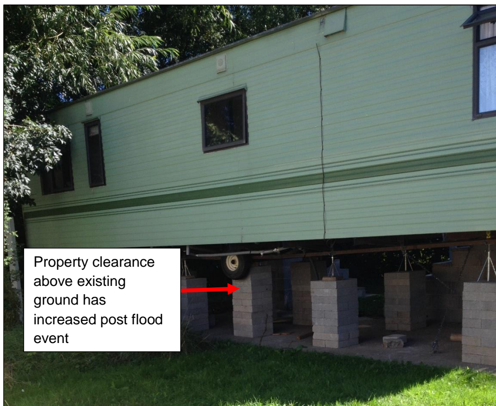
Figure 3.12 Photograph showing the increase in elevation of caravans in Knaresborough East
