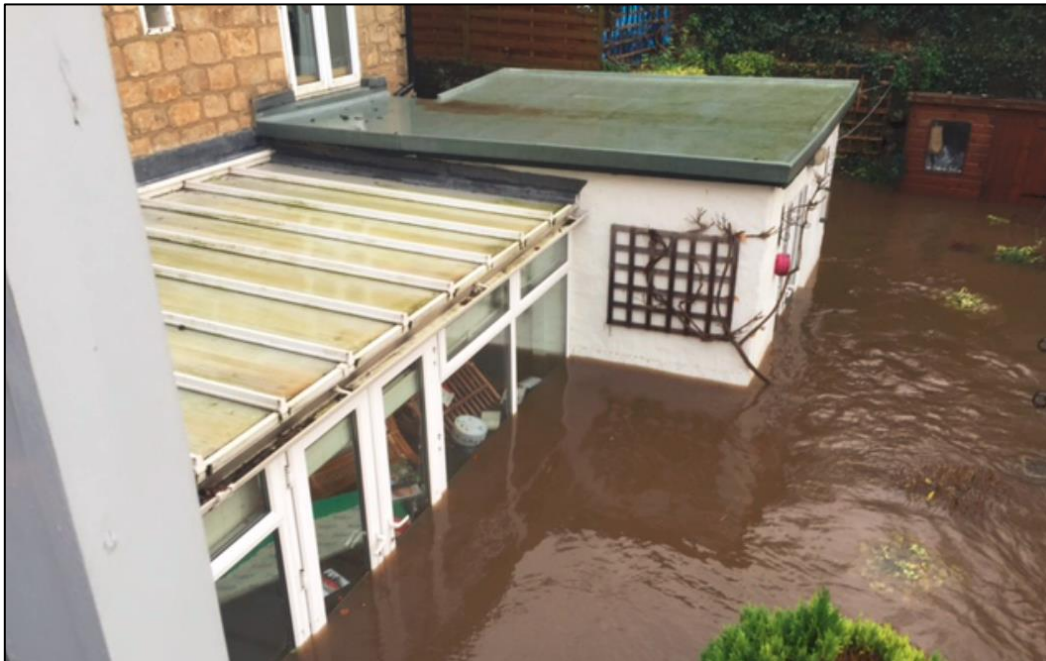
Figure 3.7 Photograph showing flooding to property in Knaresborough
