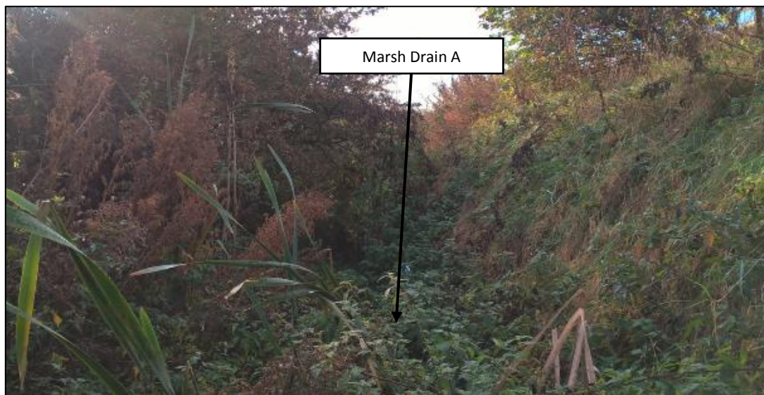
Figure 2.9 Photograph showing the current condition of Marsh Drain A
