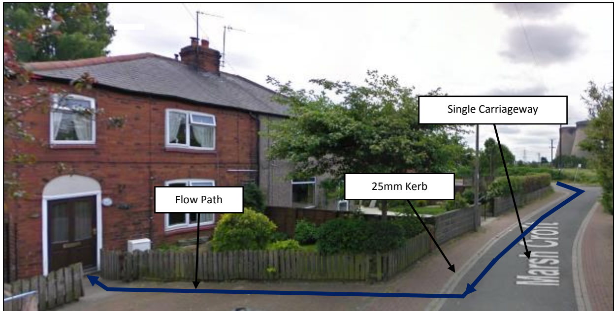
Figure 3.11 Photograph showing flow path over kerb (source: Google Maps)
