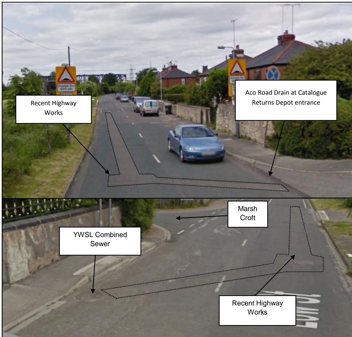
Figure 2.7 Photographs showing recent Highway works (Source: Google Maps)
